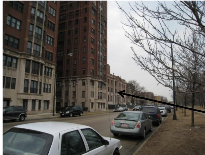
Standing southeast of the site, looking northwest at the site. Building has been demolished.
